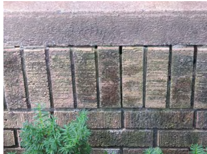
Areas of mortar loss evident in brickwork
