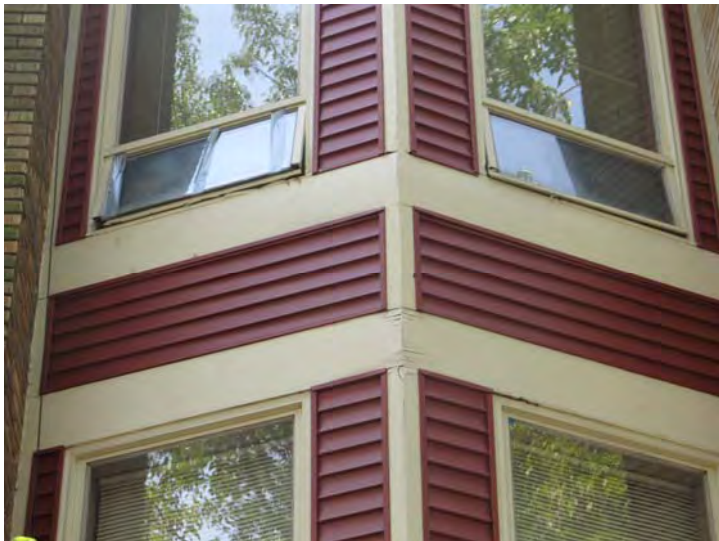
Cracks also noted in wood trim at front elevation
