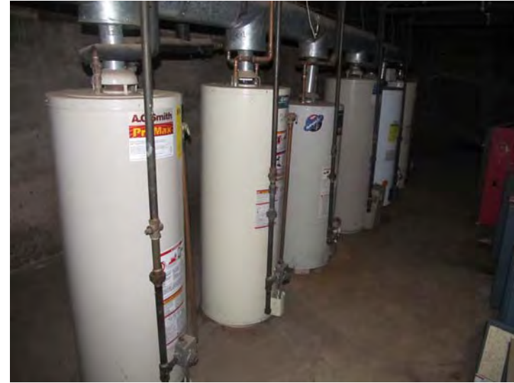
Each unit has its own natural gas-fired domestic hot water tank – Note tanks are of varying ages and brands of manufacture
