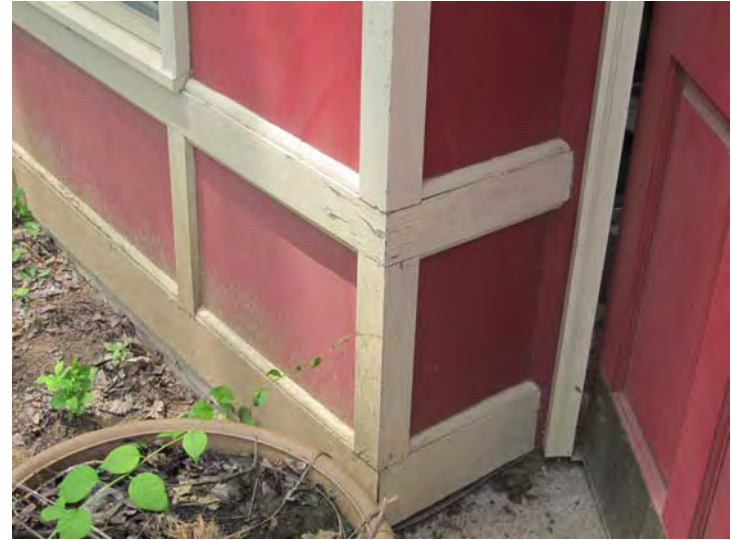
Exterior wood trim and siding at community room portion of building is in need of repair, surface preparation, and painting
