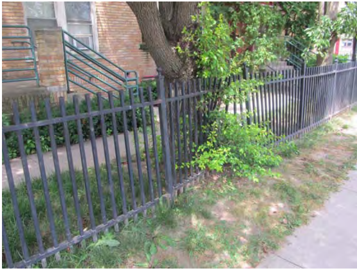
Painted iron fencing along public sidewalks is in need of minor repairs and painting
