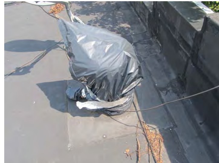
Wind driven turbine vent fans at roof level vary in condition with some being offline at the present time
