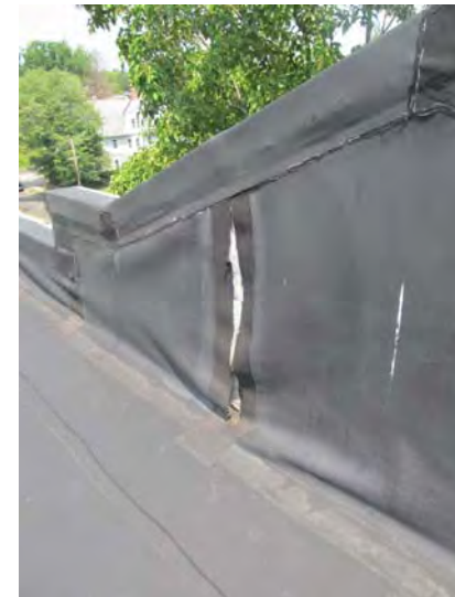
Open seam in membrane covering at back side of parapet wall
