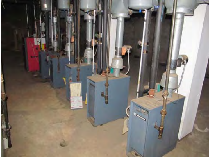
Each unit has its own boiler for production of hydronic heat – Most boilers are original and at or near the end of their expected useful service lives
