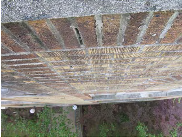
View of front elevation looking downward from roof – Note joint with missing mortar and other areas where mortar is starting to fall out of joints
