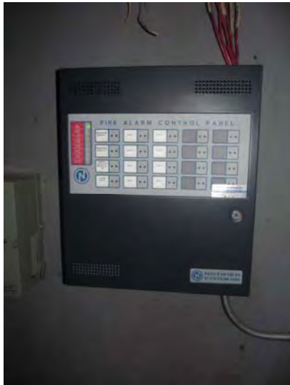
Original fire alarm control is at the end of its expected useful service life
