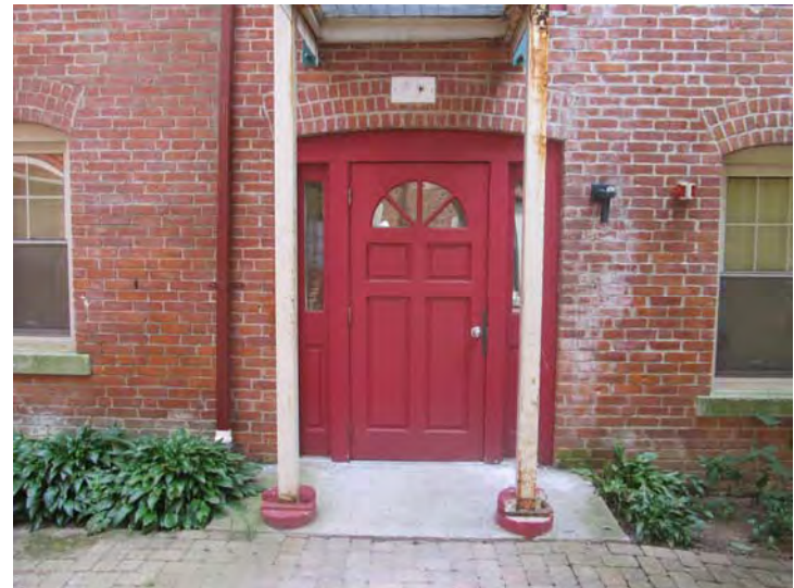
Typical common entry door – Serviceable but nearing the end of their expected useful service lives
