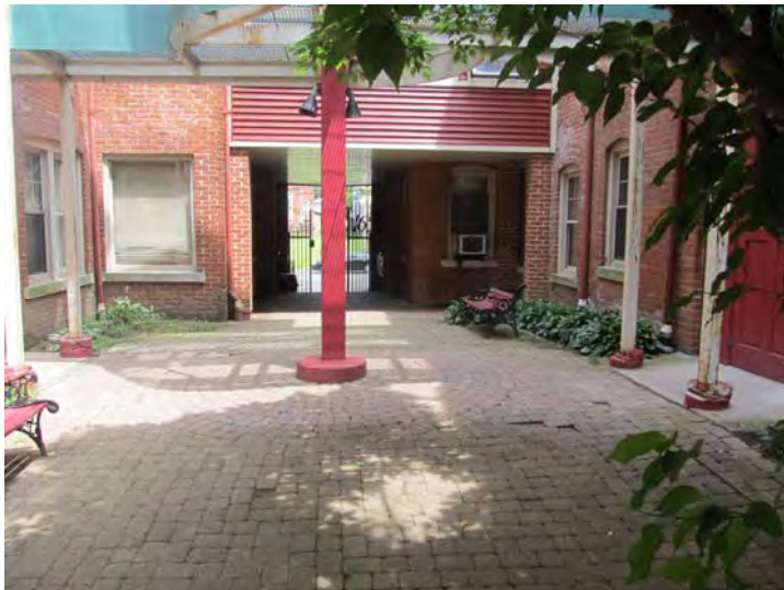
Landscape paver walkway/courtyard surfaces exhibit wear and deterioration at some locations
