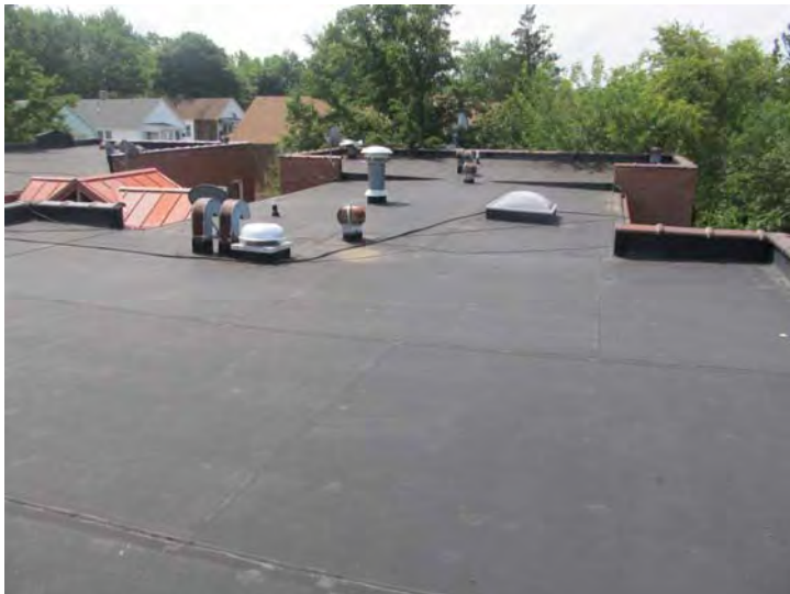
Adhered membrane roof covering is at the end of its expected useful service life
